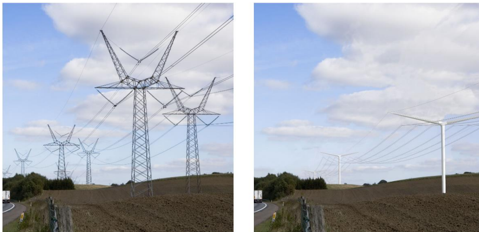
Figure 1: Conventional high voltage tower, left, comparing to the innovative composite Pylon by BYSTRUP, right. [2]
